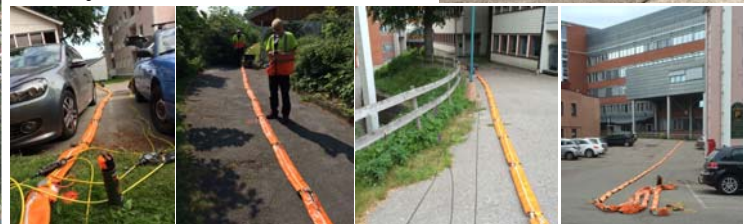
Fig. 3: Seismic data acquisition along the hospital extension area within ongoing traffic and hospital operation business. Precise positioning gained to a major challenge during seismic and drilling surveys in order to map the bedrock topography below surface.
